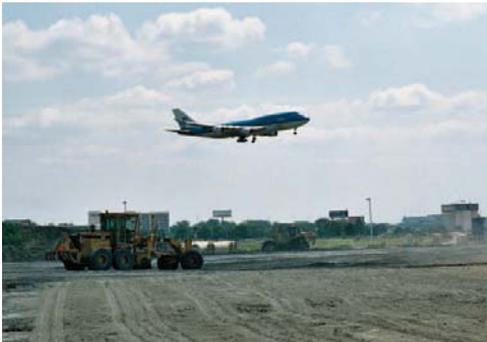
**As part of a \$15-billion program at O'Hare Airport, Lafarge supplied 100,000 tons of class C fly ash to help stabilize the soil under an extended runway.**
