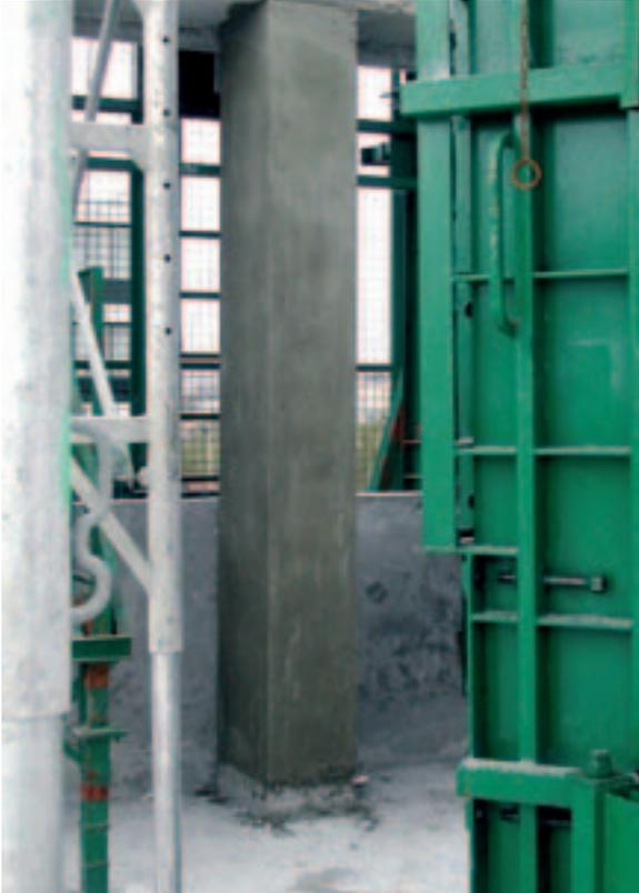
Chronolia™ concrete uses advanced technology allowing for easier placement than that of conventional concrete.\* Workability ranges from 90 to 120 minutes from batching with the benefit of high early strength which enables improved turnaround time and productivity.
