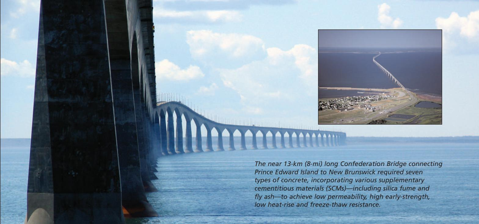
The near 13-km (8-mi) long Confederation Bridge connecting Prince Edward Island to New Brunswick required seven types of concrete, incorporating various supplementary cementitious materials (SCMs)—including silica fume and fly ash—to achieve low permeability, high early-strength, low heat-rise and freeze-thaw resistance.
