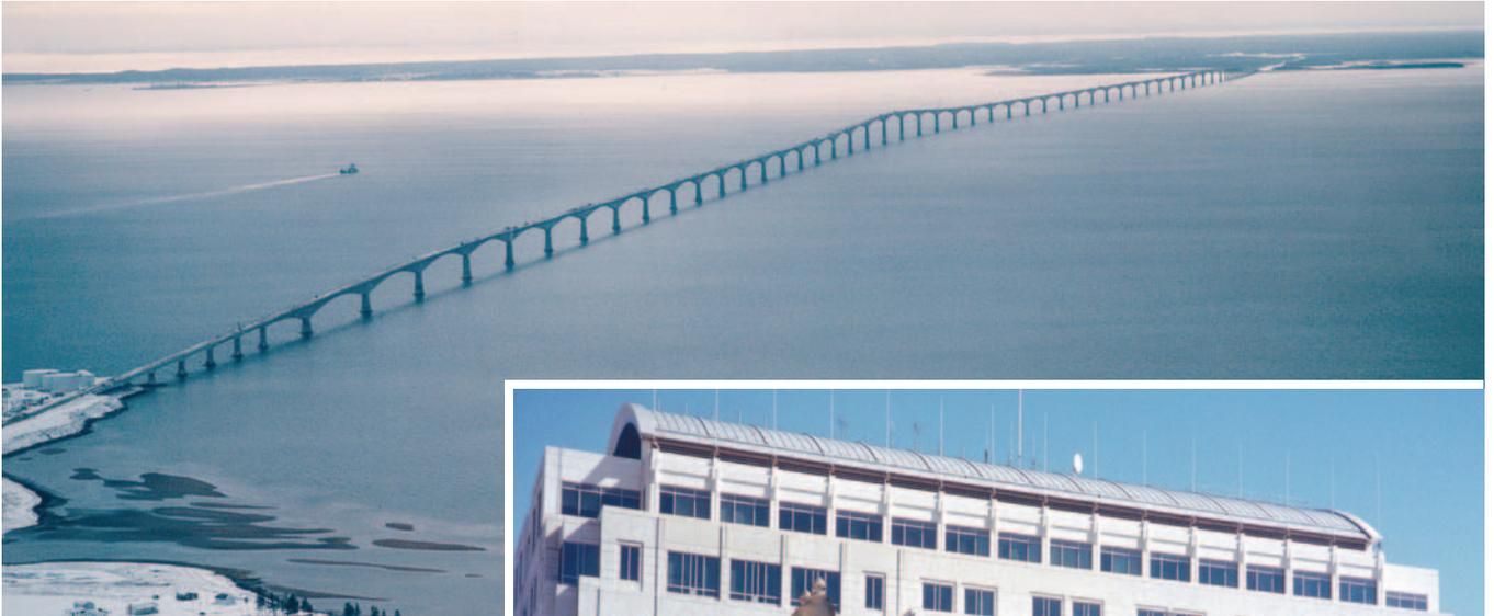
The 8-mile-long Confederation Bridge connects Prince Edward Island with New Brunswick in Eastern Canada. Seven types of concrete incorporating various SCMs — including silica fume and fly ash — were required to achieve low permeability, high early-strength, low heat rise, and resistance to freezing and thawing.
